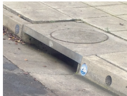
Storm drain catch basin, curbside
