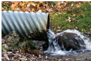
Storm drain outfall
